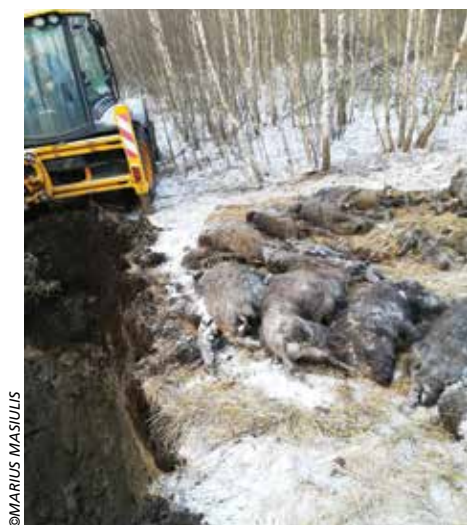
Photo 18 Trench burial needs the use of an excavator
